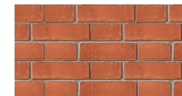
Flemish bond brick pattern used in the upper floors above the stone banding and commercial facades
