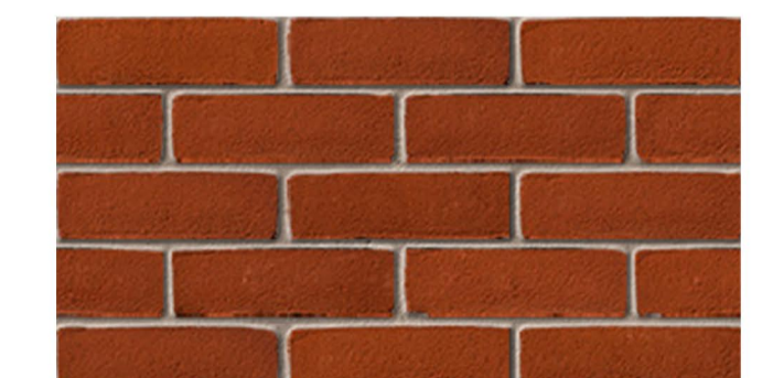
Feature brick colour used to create visual pattern within the commercial frontage
