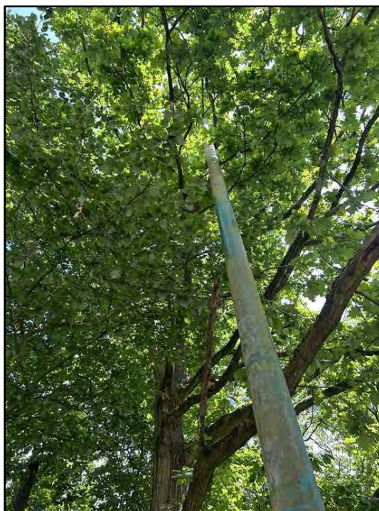
Lighting Column within tree canopy
